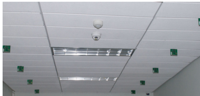
Fig 1 – Motes attached to ceiling
